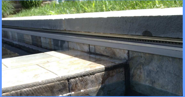
Bluestone with Encapsulated Guide
