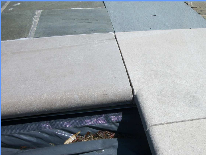
Limestone with Screw-on Guide
