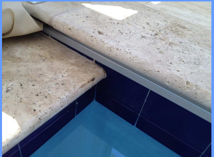
Travertine with Encapsulated Guide
