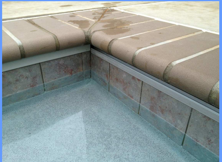
Brick with Encapsulated Guide
