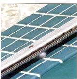
Note spacer under guide. Turn so that corner is pointing away from guide. This allows water to flow around it & under guide
