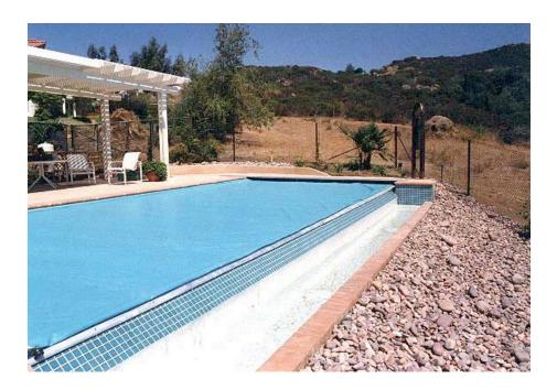
Place Top guide on tile between 2-3 inches from the top on the 45 degree slope of the outside edge of the vanishing edge.
