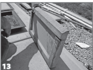
13 The trays were designed so the middle section of the lid will be thinner to reduce the weight of the lid section.
