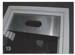
Lower the lid lock bracket so the slots on the front side of the bracket slide over the remaining pem studs in the anchor plates.
