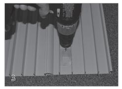
With the backing plate in position, use a drill with a 1/4" drill bit to drill through the small hole in the backing plate and through the lid panel.
