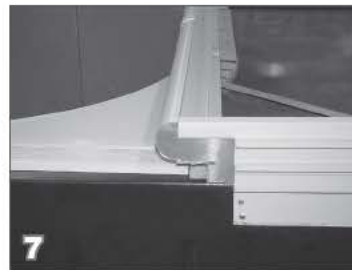
7 If using a Coverstar Encapsulation with coping, install the transition pieces that will fit between the riser panel and the encapsulation/coping.
