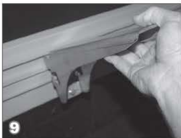
9 Install the lid brackets into the riser along the back of the housing. Place a level on the brackets and level them by adjusting the bolt at the bottom of the bracket.
