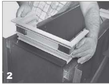
2 Place the preassembled boxed riser ends (A2410) at each end of the housing.
