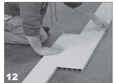
12 Slide the two sections of lid together. Slide the descenders on the front side of the lid. Position the lid in so it rests on the lip of the riser and on the lid brackets. Make sure the lid is in place when the concrete is poured. The lid can be masked off or turned upside down to keep it clean during the concrete pour.
