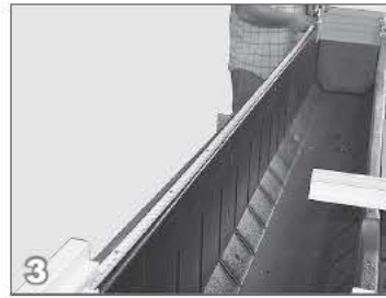
3 Measure across the back of the housing between the boxed ends. Cut a length of the riser (X0944) to fit in this opening.
