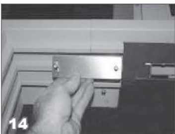
14 Position the anchor plate into the top channel of the riser by inserting it at an angle so the top of the anchor plate goes into the channel first, and then move the bottom of the plate into the channel. Repeat this process for the other anchor plates.
