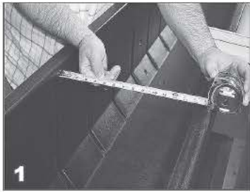
1 Check the inside width of the cover housing. Make sure it matches the width of the flush lid kit that was ordered.
