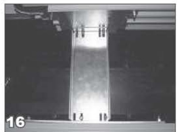
16 Install the cross braces over the pem studs in the QuickAttach brackets at both the motor and non motor ends of the housing. These cross braces will maintain the correct width between the QuickAttach mechanism mounting plates during the concrete pour. Secure using 1/4 - 20 nylock nuts. These cross braces will be removed when the mechanism is installed.
