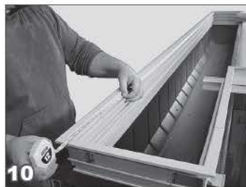
10 Measure from the inside of one riser boxed end to the other in order to determine the total lid length. Cut the lid panels to this length.
