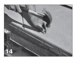
Remove the lid and hammer the plastic anchors (A1706) into the holes.
