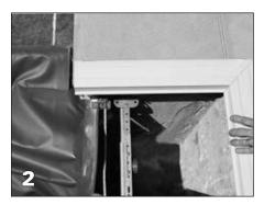
Set the lid end supports (A2429) in the ends of the housing in order to get an accurate measurement for the lid panels.
