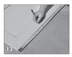
With the lid completely assembled, set it over the housing. Now mark and drill holes through the lid hinge approximately every 18 inches. Drill the holes into the deck through the holes in the lid hinge
