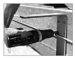
Attach the brackets of your choice (ordered separately) to the back wall of the housing 1 in below the top of deck.
