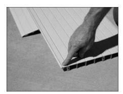
The hinge attachment should be flush with the end of the lid and the lid hinge is offset from the end.
