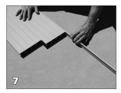
Slide the lid panels (X0048) and C-cap (X0053) together.
