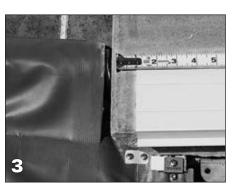
Mark and cut the front side of the lid end supports leaving at least 1 in of flat surface between the coping edge and the lid end support.
