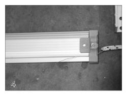
Feed the rope into the water side channel of the track with the wire extending out the side of the track. Use the wire to pull the rope down the length of the track towards the end of the pool.
