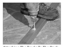
Attaching The Tracks To The Deck Place the tracks into position on the deck in the marked positions. Make sure that the tracks run completely straight on both sides of the pool. Drill through the pre-drilled holes into the deck. Drill at least 3" deep.
