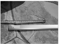
Extend the tracks 18" past waterline. Center the pool shape between the pool tracks where possible. Measure and mark the track length on the deck. Use a chalk line to mark the track location.
