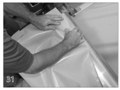
Attaching The Cover & Bonding Wire At the motor end, attach the tail of the cover and the bonding wire to the roll-up tube using 1/2" tek screws (26). Make sure the webbing continues straight as it travels from the track to the roll-up tube. Attach the cover and bonding wire to the roll-up tube on the non-motor end in the same manner. Webbing should roll up completely off the tube.
