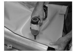
The first two screws need to be 3" from the end of the tube. Distribute the slack of the cover evenly across the length of the tube. Secure the cover to the roll-up tube using tek screws every 2-3ft. When attaching the cover to the tube, do not use folds or pleats.
