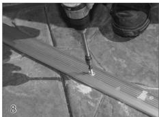
Complete the fastening of all track screws flush to the top of the track. Clean concrete dust from track and pulley end cap. Make sure ALL screws are flush with the top of the tracks.
