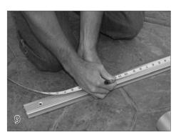
Cutting The Tracks To Length With tracks extended at least 18" past the waterline at the opposite end of the pool, cut the tracks so they extend 18" past the waterline at the mechanism end.
