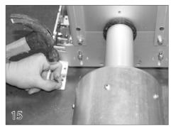
Use the 1 1/2 hex head screws (35) and anchors (25) provided to secure the motor end and non motor end to the deck.
