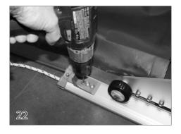
Install a stop on the end of the track near the mechanism to keep the cover from retracting too far. Secure the stop to the deck using the screws (19) and anchors (25) provided. Run the key switch in the uncover position to roll the cover up on the roll-up tube. Check the cover to be sure it rolls up evenly.
