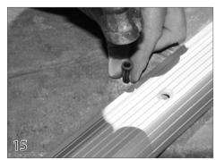
Move the tracks to the side to expose the holes in the deck. Tap the plastic anchors (25) into each hole.
