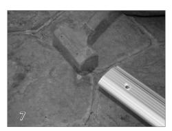
At one end, use a rubber mallet to tap the track sections together.
