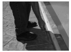
Feed the rope into the back channel of the track, then pull the rope down the back side of the track toward the cover housing.
