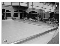
Running The Cover Over The Pool Run the cover over the pool being careful to prevent it from binding in the guide feeds by lifting the cover and helping it into each track the first time.
