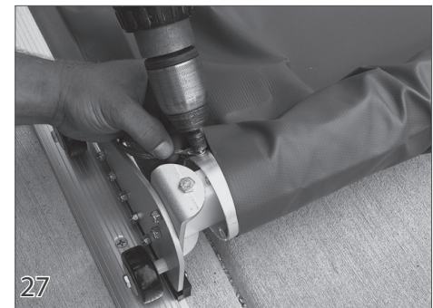
27 Connect the bonding wire that is attached to the front corner of the cover to the leading edge bar using a tek screw (49). Be sure the screw doesn't interfere with the leading edge insert.
