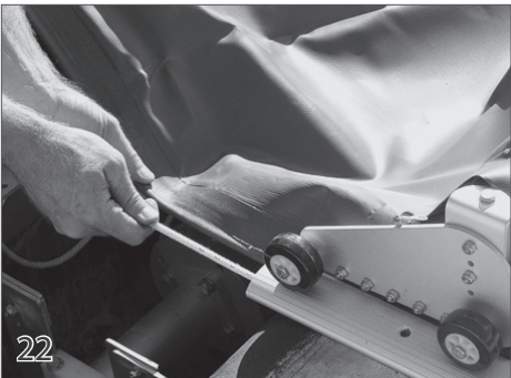
22 Feed the wheel assembly and cover into the track. The slider on the front of the wheel assembly will lock into the track.
