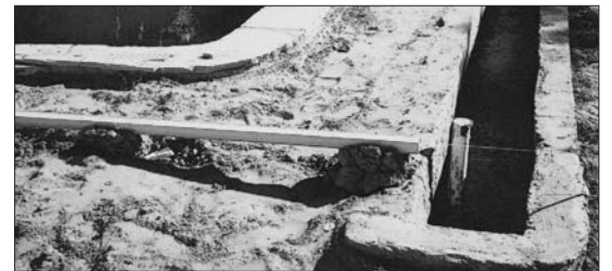
(4.b.) Housing in place mounted on gunite piles ready for deck pour.
