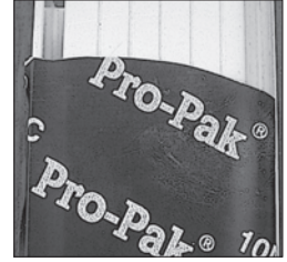
(3) Guide protected by 2" 10 mil plumbers tape
