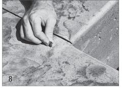
Insert plastic anchors (33) into the holes and tap with a hammer so they are flush with the deck. Fasten the lid to the deck with #12 pan head screws (26).
