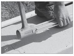
Lay the sections of guide on the deck and tap them together using a rubber mallet so the center splice and splice pins interlock with each section of guide. It's important that, the splice is tight together so there is not a gap from one guide to the next. Slide pulley end cap (15) into the end of the guide at that is at the opposite end of the pool from the mechanism.
