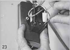
Insert the RED DIRECTIONAL WIRE into terminal B1, and tighten the screw.
