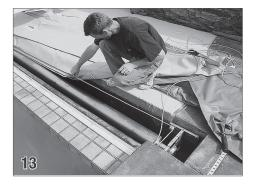
Pull the rope along the back of the housing to the motor side.
