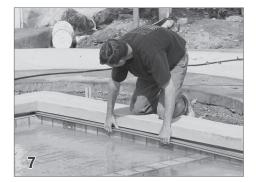
**Encapsulated Underguide (optional)** If encapsulation is being used, the guide is normally installed during the cover installation. (See cover installation section page 10, step 9).
