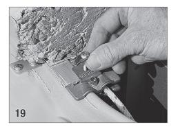
Place a guide feed over the end of the guide, place a bonding lug (25) on top of the guide feed. Insert a  $10-32 \times 1 3/4$ " screw (42) through the lug and guide feed.
