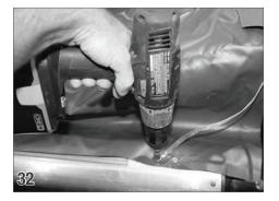
Lay the bond wire on top of the cover fabric. Secure it to the roll up tube using a tek screw (32). Distribute the slack of the cover evenly between each screw across the length of the tube. Secure the cover to the roll-up tube using tek screws (32) every 2-3ft. When attaching the cover to the tube, **do not use folds or pleats**.
