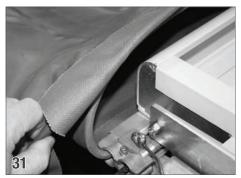
Attaching The Cover & Bonding Wire Make sure the webbing continues straight as it travels from the guide to the roll-up tube. Attach the cover to the roll-up tube using tek screws (32). The first screw on each end of the tube needs to be 3 inches from the end of the tube. As the cover rolls up on the tube, the webbing should roll up completely off the tube.
