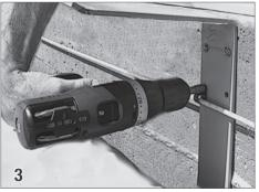
Secure the brackets to the back wall of the housing using #12 x  $1\frac{1}{2}$  "hex head (34) screws. Mount a rope loop (30) on one screw of each of the brackets. This will keep the rope running straight along the back of the housing.
