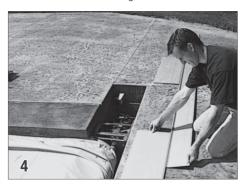
**Assembling The Aluminum Lid** The aluminum lid will come with each section cut to length. Assemble the lid by sliding the hinge onto the main section of lid.
