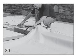
**Running Out The Cover** Run the cover over the pool being careful to prevent it from binding in the guide feeds by lifting the cover if necessary.
