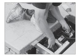
**Positioning the Mechanism** Lower the assembled mechanism and tube into the housing and place it roughly in the position that it will anchored.
