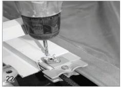
Drill through the center of the encapsulation and guide. Insert a  $10-32 \times 1$  3/4 screw (42) and nylock nut (29). This step is very important. This will prevent the guide from sliding into the cover housing duirng the operation of the cover system.
