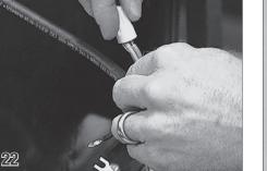
Attach the other leg from the indicator light and the BLUE DIRECTIONAL WIRE into terminal A1, and tighten the screw.
