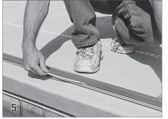
Hold the rope outside the guide to pull the rope down the length of the guide toward the end of the pool.
