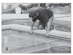
**Install Guide in the Encapsulation** Starting at one end, lift the guide so it will interlock with the encapsulation. Make sure the guide extends 1" into the housing.
