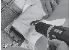
Position the fabric on the leading edge so it is in line with the leading edge support bracket. Secure with a tek screw (32) on the back side of the leading edge. Be sure the screw does not interfere with the leading edge insert.
