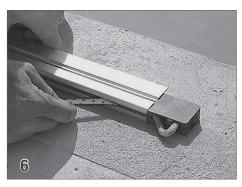
Now, feed the rope through the pulley assembly. Insert the pulley into the end of the guide.
