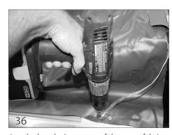
Lay the bond wire on top of the cover fabric. Secure it to the roll up tube using a tek screw (32).
