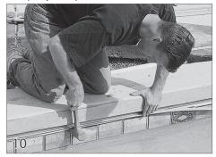
Insert and tap the spacer into place underneath the track along the entire length of the track. Do this along both sides of the pool. The spacer needs to end at the inside edge of the cover box.
