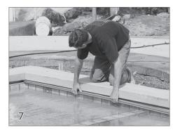
When encapsulation is being used, the track is normally installed during the cover installation. (See cover installation section page 10, step 9).
