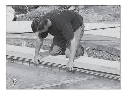
Install Track in the Encapsulation Beginning at the shallow end of the pool, insert the track into the encapuslation. Lift the track so the tongue and groove between the track and encapsulation will interlock. Make sure the track extends 1" into the housing.
