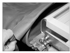
Attaching The Cover & Bonding Wire Make sure the webbing continues straight as it travels from the track to the roll-up tube. Attach the cover to the roll-up tube using tek screws (32). The first screw on each end of the tube needs to be 3 inches from the end of the tube. As the cover rolls up on the tube, the webbing will be rolling up over the cone.
