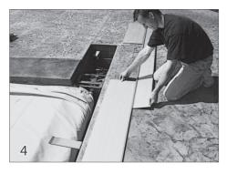
Assembling The Aluminum Lid Assemble the lid by sliding the hinge onto the main section of lid.
