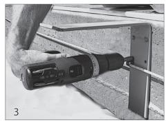
Secure the brackets to the back wall of the housing using  $\#12 \times 1\frac{1}{2}$  "hex head screws( 34). Mount a rope loop (30) on one screw of each of the brackets. This will keep the rope running straight along the back of the housing.
