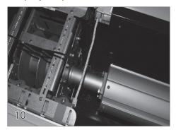
Align the mechanism on the motor side first by using a length of rope and extending it from the back side of the cover track to the pulley to make sure the rope will feed directly into the pulley.
