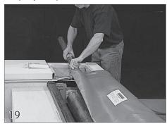
Inserting the Leading Edge Tube Lay the front of the cover across the bond beam. Slide the leading edge tube through the loop on the front of the cover. If the leading edge tube will remain exposed, slide the tube on to the bead on the front of the cover.
