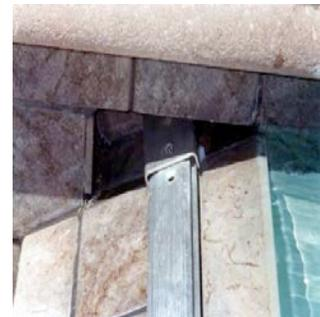
If end of pool has a raised bond beam, it must be notched for the end pulley
