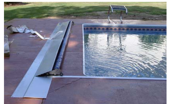
Installed pool cover system under standard aluminum lid..
